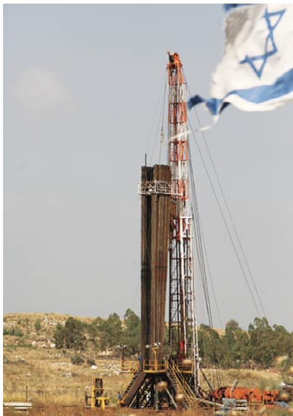
THE DRILL SITE Zion's well rises from fertile kibbutz land.
